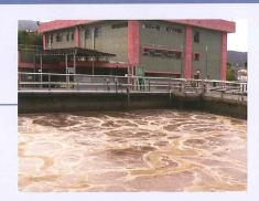
The thickened primary sludge and SAS are pumped into the sludge digesters for aerobic digestion.
