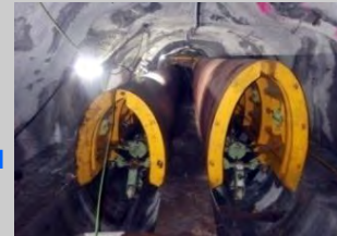
預製的鋼模板 Prefabricated Steel Shutter Formwork
