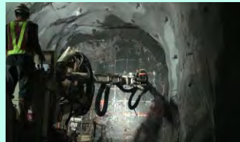
鑽炮孔 Drilling Blast Holes
