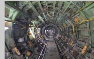
伸縮式模板 Telescopic Formwork
