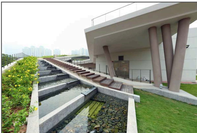
Kowloon City Sewage Pumping Station No.1
