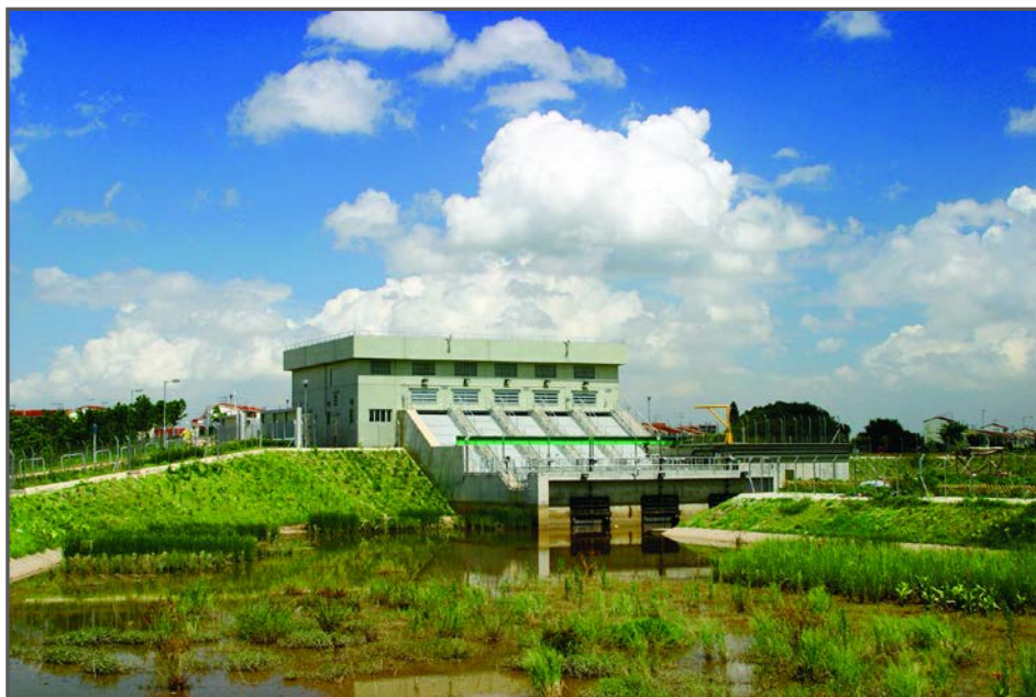
Chuk Yuen Tsuen Stormwater Pumping Station
