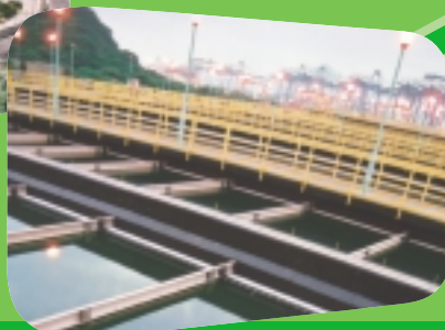
污染物在沉澱池沉澱 Pollutants settling in sedimentation tanks
