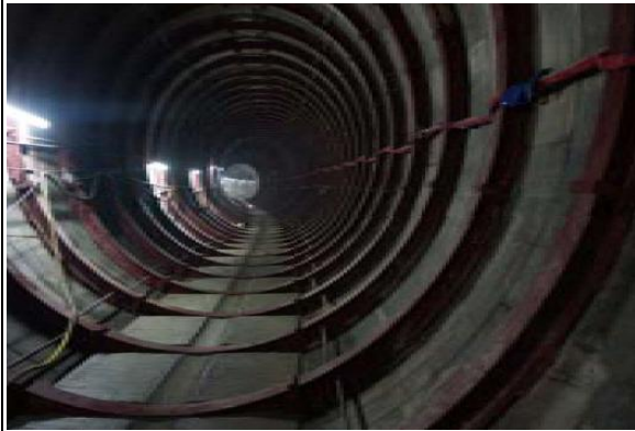
Main Tunnel of Lai Chi Kok Drainage Tunnel
