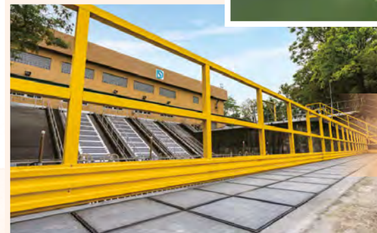
設於新田雨水泵房的可踏式太陽能發電系統 Steppable Photovoltaic System at San Tin Stormwater Pumping Station
