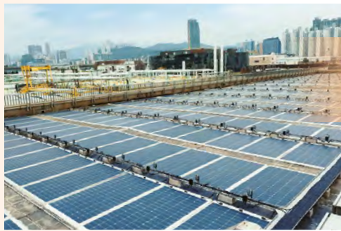
設於西北九龍基本污水處理廠的柔性單晶硅太陽能發電系統 Flexible Monocrystalline Photovoltaic System at North West Kowloon Preliminary Treatment Works
