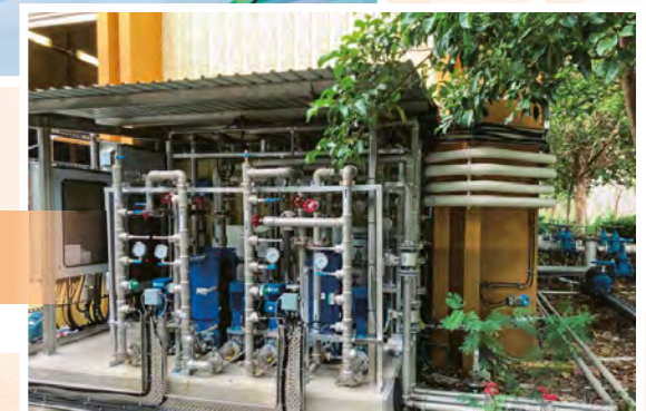
排放水水冷式空調系統 Effluent Cooling Air Conditioning System
