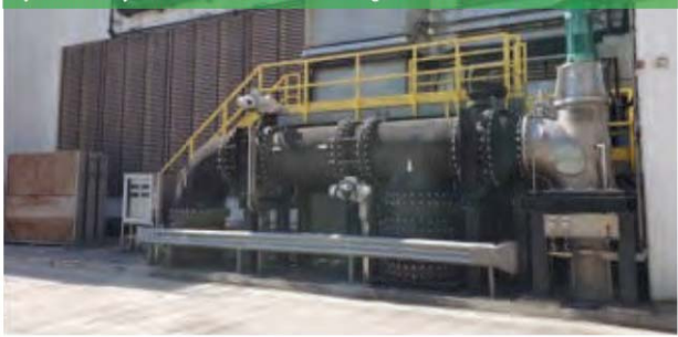
昂船洲污水處理廠的水力渦輪系統 Hydro-turbine system at Stonecutters Island Sewage Treatment Works
