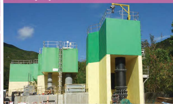
新建的加壓污水管及漩渦室 The new sewage rising main and vortex chamber
