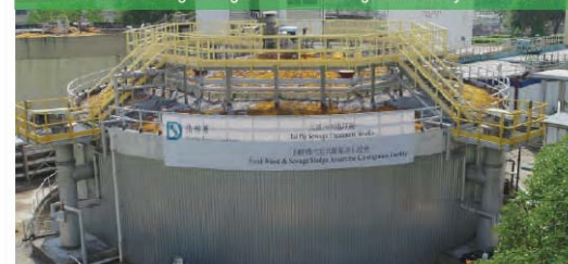
大埔污水處理廠內的廚餘、污泥共厭氧消化設施 Food Waste and Sewage Sludge Anaerobic Co-digestion Facility at Tai Po STW
