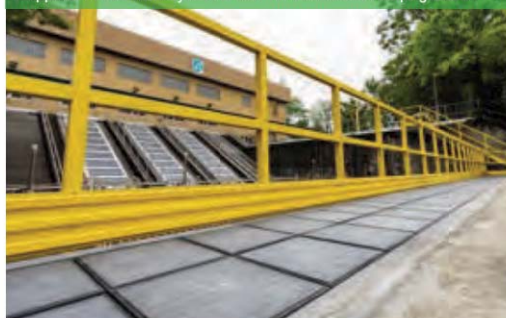
設於新田雨水泵房的可踏式太陽能發電系統 Steppable Photovoltaic System at San Tin Stormwater Pumping Station
