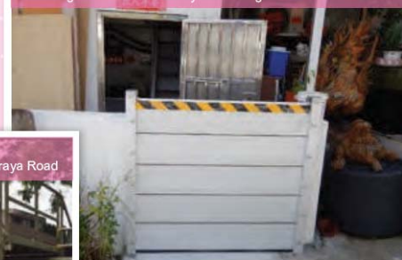
協助受風暴潮影響的住戶安裝擋水板 Assisting residents affected by storm surge to install flood barriers
