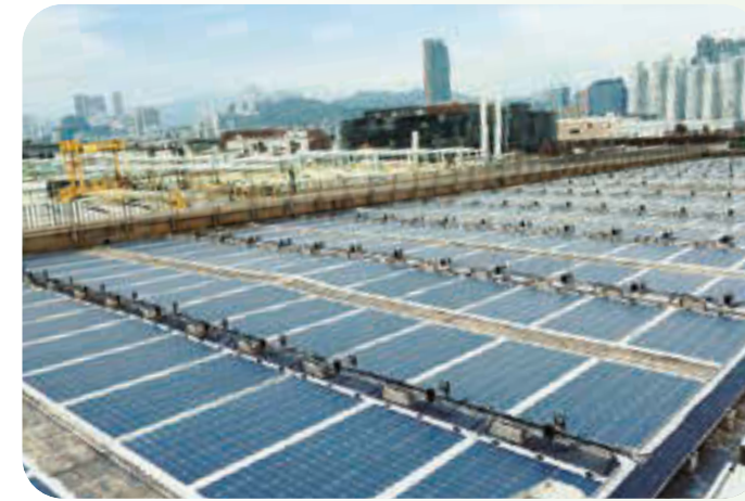
◀ 設於西北九龍基本污水處理廠的柔韌單晶硅太陽能發電系統 Flexible Monocrystalline Photovoltaic System at North West Kowloon Preliminary Treatment Works
