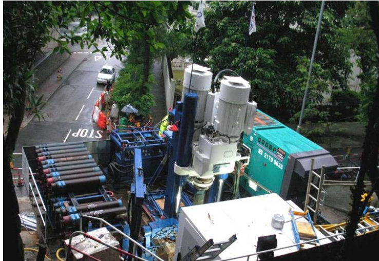
Figure 8 Raise boring equipment setup at Intake location
