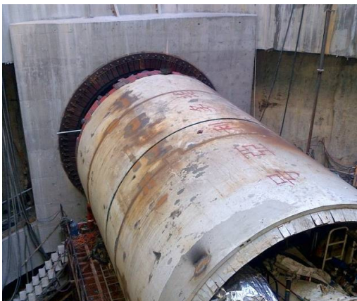
Photo 1 – Collar and Mechanical Seal at TBM Launching
