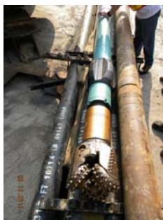
Fig.14: Tri-cone Bit for Pilot Hole Drilling
