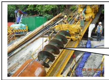
Fig. 5 Pipe Ramming of 48" Steel Casing
