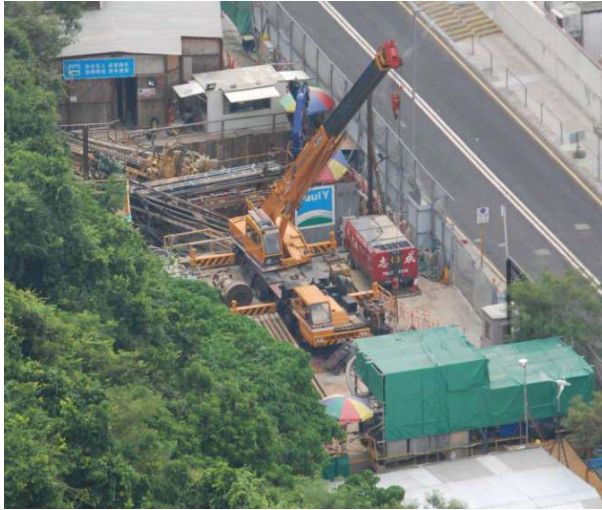
Fig. 8: HDD Plant & Equipment Set Up at Aberdeen Entry Point
