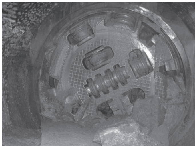
Figure 32 – TBM Breakthrough in Receiving Permanent Shaft
