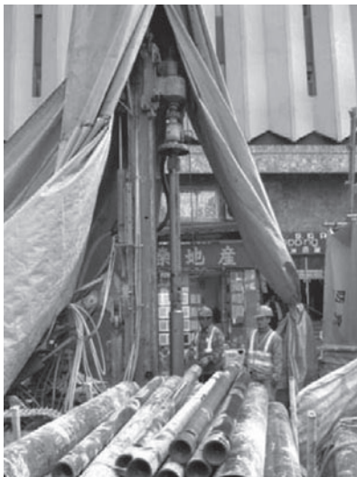
Figure 4 – Pipejacking Works in Progress
