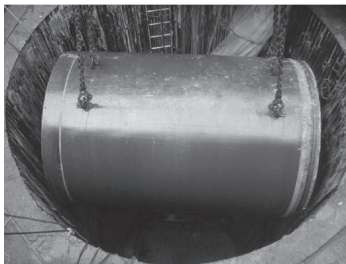
Figure 33 – Lifting-up of the Longest Machine Can of TBM from Receiving Shaft
