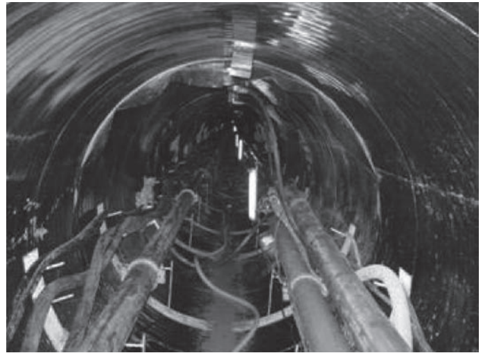
Figure 21 – Typical Condition of a Jacked Pipeline
