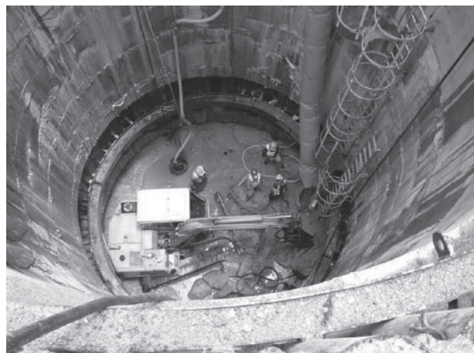
Figure 5 – Construction of 5.5 m Diameter Concrete Ring Wall
