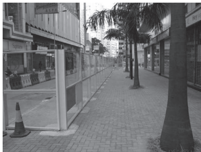
Figure 24 – Fully Transparent Hoarding in a Work Site
