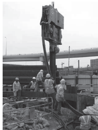
Figure 3 – Sheetpiling Works in Progress
