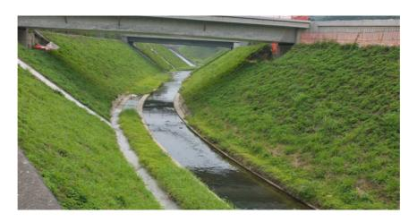
FIGURE 40 GRASSED CELLULAR CONCRETE PAVING AT MA WAT RIVER
