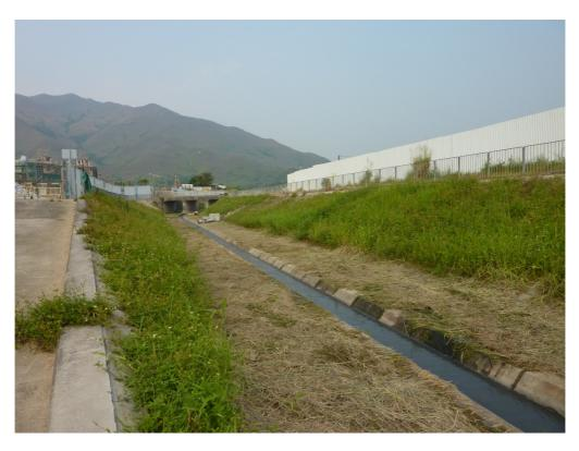
FIGURE 9 DRY WEATHER FLOW CHANNEL AT TAI KONG PO
