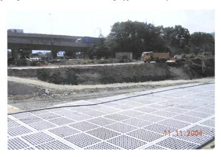
FIGURE 32 GRASSED CELLULAR CONCRETE PAVING AT YUEN LONG BYPASS FLOODWAY (DURING CONSTRUCTION)
