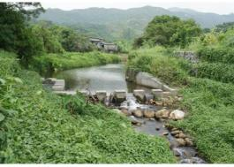
FIGURE 18 FISH LADDER AT HO CHUNG RIVER (LEFT) AND PAK NGAN HEUNG RIVER (RIGHT). FOR PAK NGAN HEUNG RIVER, THE FISH LADDER MAY BE FURTHER IMPROVED THROUGH THE USE OF NATURAL SUBSTRATES AND SLOPING GRADIENTS FOR THE EMBANKMENTS AT THE WEIR UPSTREAM TO FACILITATE ANIMAL PASSAGE.
