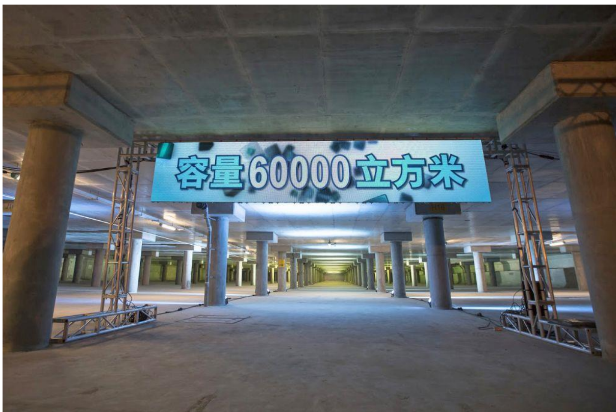
FIGURE 15 HAPPY VALLEY UNDERGROUND STORMWATER STORAGE SCHEME
