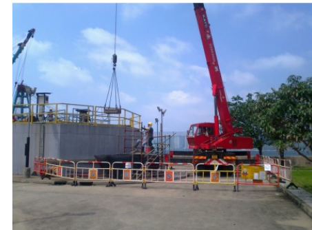
Removal of scum from Drop Shaft at Chai Wan Preliminary Treatment Works
