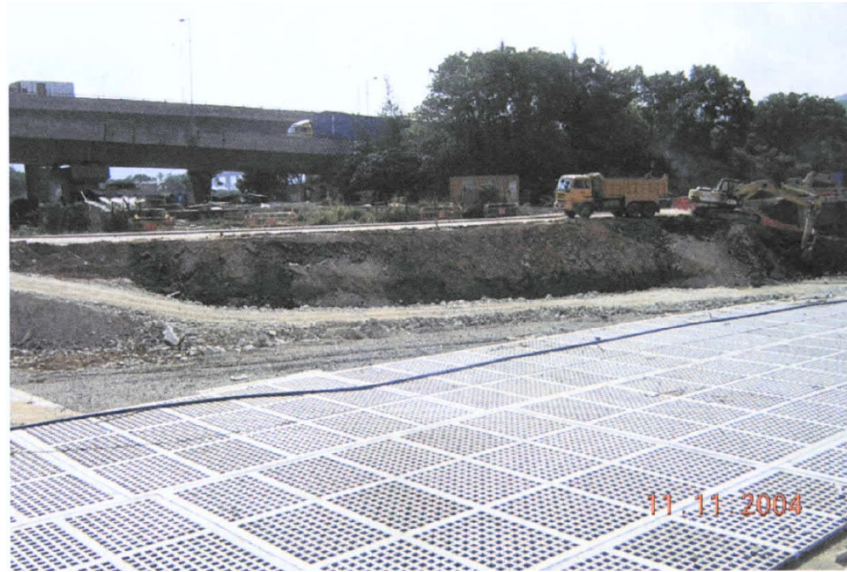
FIGURE 35 GRASSED CELLULAR CONCRETE PAVING AT YUEN LONG BYPASS FLOODWAY (DURING CONSTRUCTION)
