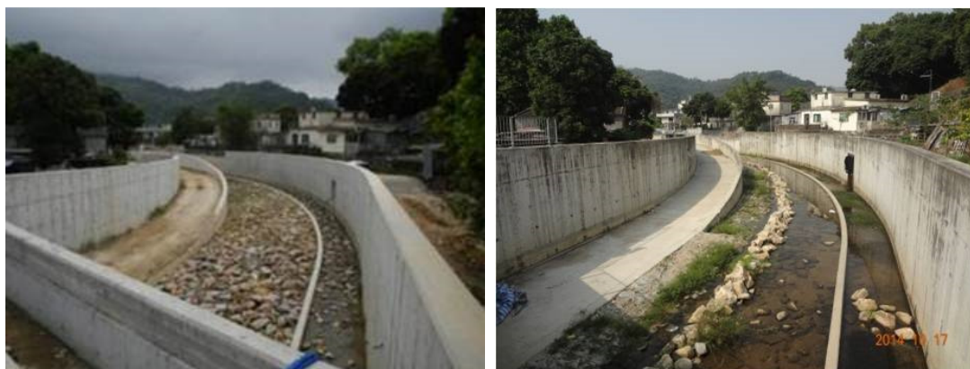
FIGURE 28 RIP-RAP BEDDING IN KAU LUNG HANG. THE ORIGINAL DESIGN OF RIP-RAP BEDDING (LEFT) AND MODIFICATION OF THE RIP-RAP BEDDING IN THE CHANNEL DURING DRY SEASON (RIGHT)
