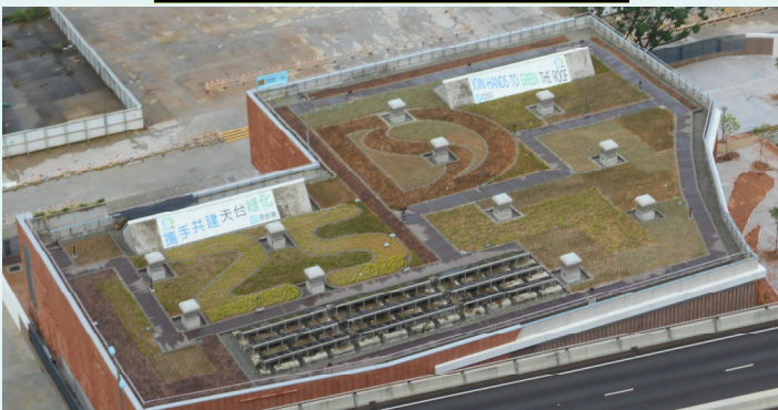
Green Roof of Flow Interception Station
