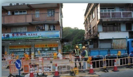
重新鋪設街燈線路及道路 Laying of road lighting cables & construction of footway
