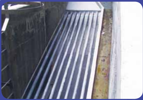
Surface runoff interception point at existing stream course and culvert
