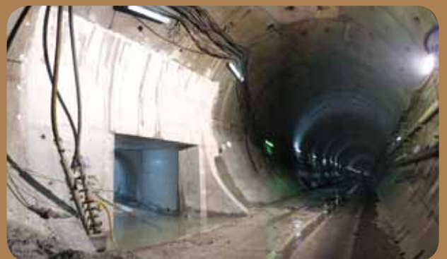
Junction of the main tunnel and adit tunnel - under construction
