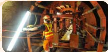
Adit lining works in progress
