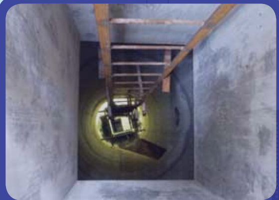
A shaft to allow surface runoff to fall from ground level down to the adit level
