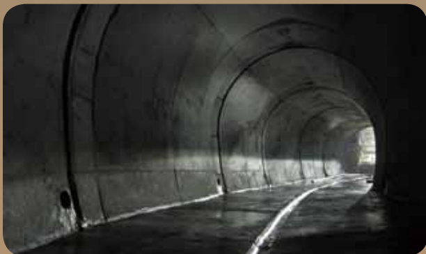
Adit tunnel to convey stormwater to main tunnel
