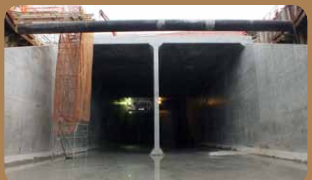
The discharge point of stormwater from the main tunnel - under construction
