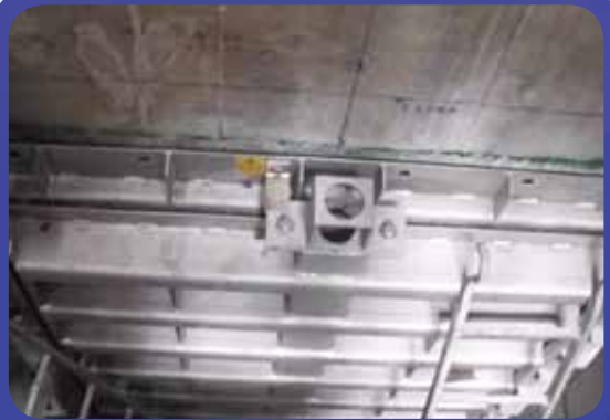
Penstock is the gate to prevent surface runoff entering the tunnel during maintenance
