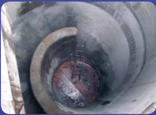
Surface runoff entering the dropshaft
