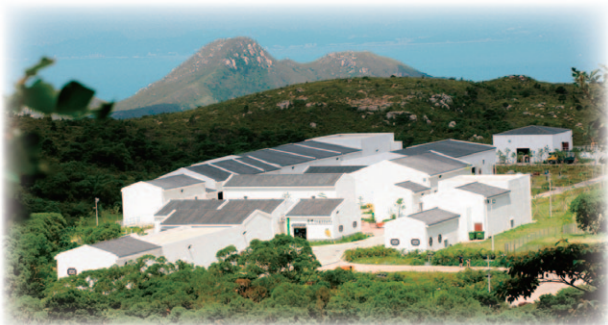
Ngong Ping Sewage Treatment Works
