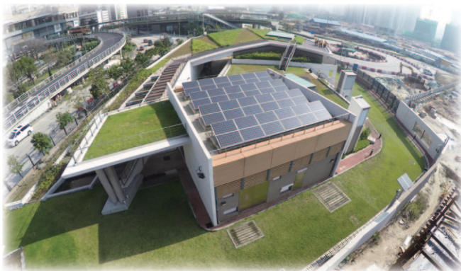
Kowloon City No.1 Sewage Pumping Station
