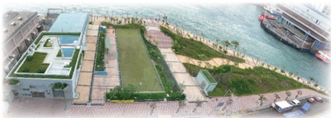
Sheung Wan Stormwater Pumping Station
