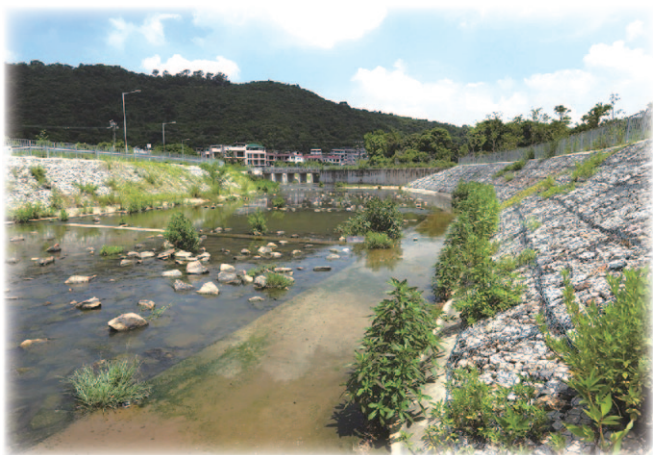
Completed Tai Po River
