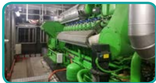
沙田污水處理廠的1.4兆瓦熱電聯供發電機 A 1.4-megawatt combined heat and power generator at Sha Tin Sewage Treatment Works
