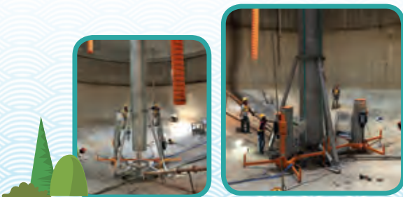
工作人員在大埔污水處理廠的指定污泥消化缸內安裝廚餘與污泥共厭氧消化新混合器 Installation of new mixer inside the sludge digester designated for food waste and sludge co-digestion at Tai Po Sewage Treatment Works
