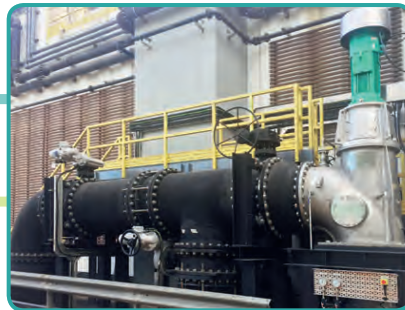
昂船洲污水處理廠的水力發電系統 Hydro-turbine system at Stonecutters Island Sewage Treatment Works
