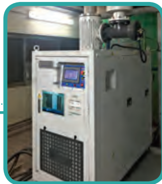
赤柱污水處理廠空氣軸承高速渦輪鼓風機 Air-bearing type high speed centrifugal air blowers in Stanley Sewage Treatment Works
