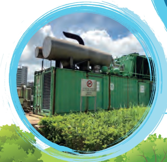
大埔污水處理廠的電熱聯供發電系統 Combined heat and power generating system in Tai Po Sewage Treatment Works
