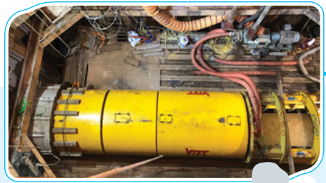
東涌污水泵房利用隧道鑽挖機進行非開挖工程 Trenchless works using tunnel boring machine at Tung Chung Sewage Pumping Station
