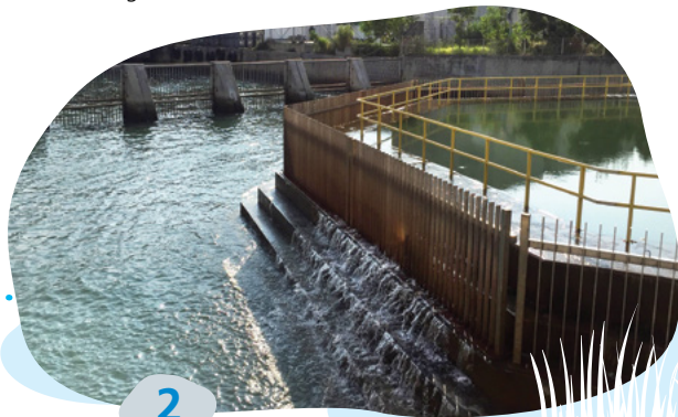
2. 荔枝角雨水排放隧道出水口 Outfall of Lai Chi Kok Drainage Tunnel
