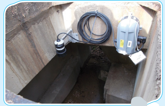
沙井內的數據收集器和超聲波傳感器能實時監測水位變化 Data loggers and ultrasonic sensors in manholes can monitor real-time water level movements
