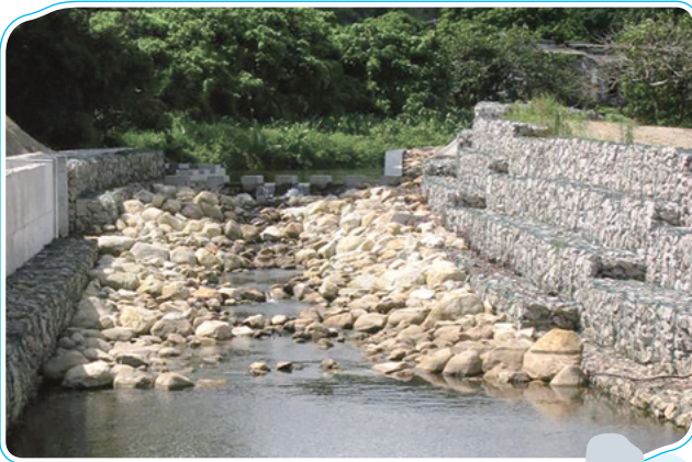
蠔涌河的魚梯由不規則的石塊和卵石形成 Randomly placed boulders and cobbles form the fish ladders in Ho Chung River
