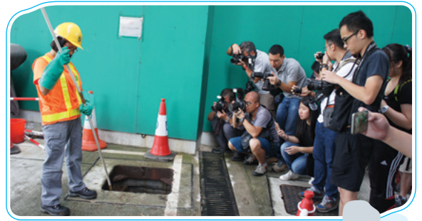
女通渠工朱運秋女士示範運用藤具清理渠道 Ms. CHU Wun-chau, female Leading Sewerman, demonstrating drain cleansing with rattan tool
