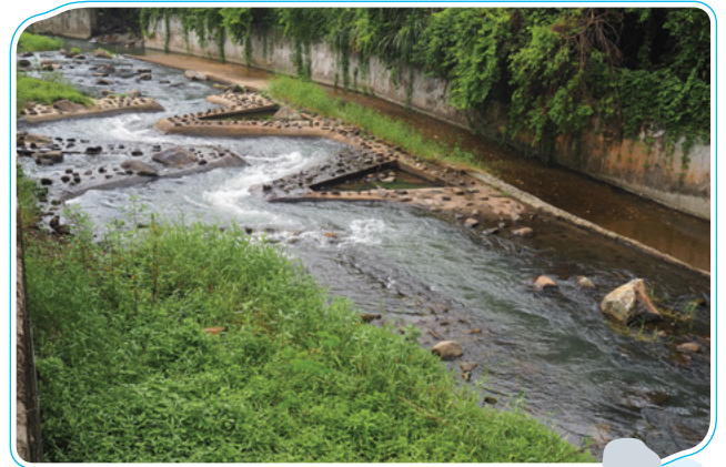
林村河上游3條「之」字型設計的魚梯，上設凹位，供魚類棲息 Three zig-zag fish ladders in Upper Lam Tsuen River designed with still water troughs to provide refuge for fish
