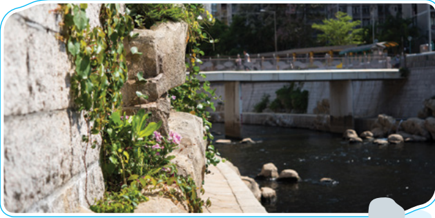
盆中設有種植空間，讓植物在石縫生長，覆蓋河堤 The artificial rock planters offer space for crevice plants to grow and cover the embankments
