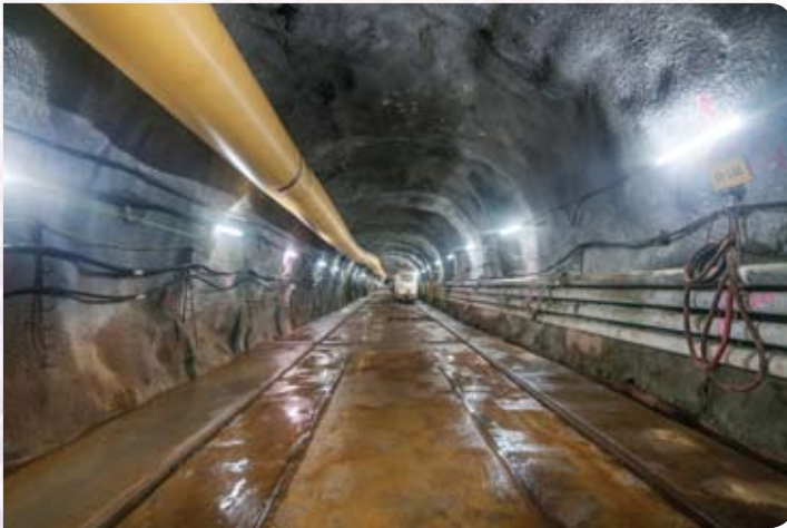
採用鑽爆方法建造的隧道 Tunnel section constructed by drill-and-blast method
