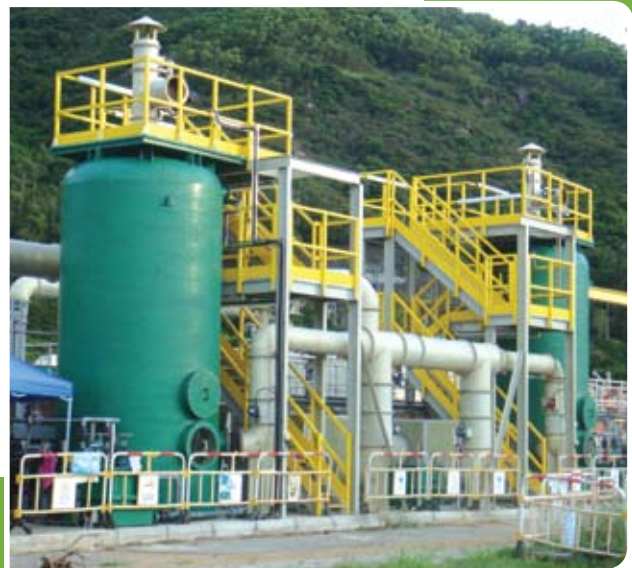
生物滴濾塔除味裝置 Biotrickling Filters
