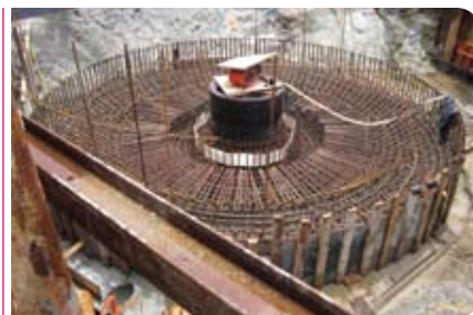
華富、香港仔及鴨脷洲基本污水處理廠現正進行幼隔篩及除砂設施建造工程 Construction of fine screen and grit trap structure at Wah Fu, Aberdeen and Ap Lei Chau PTWs is in progress
