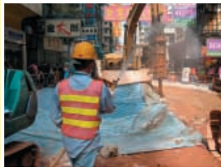
在登打士街灑水，防止塵土飛揚 Spraying of water to prevent dust at Dundas Street
