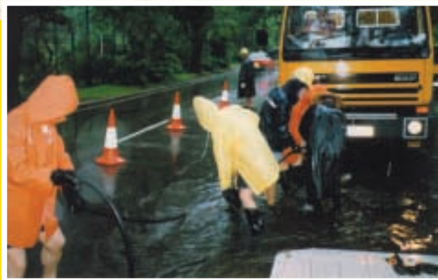
緊急清理淤塞的排水渠 Emergency clearance of blocked drain
