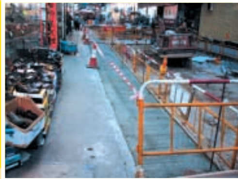
於施工期間，擴闊一段西貢街的行人路 Temporary widening of footpath in Saigon Street
