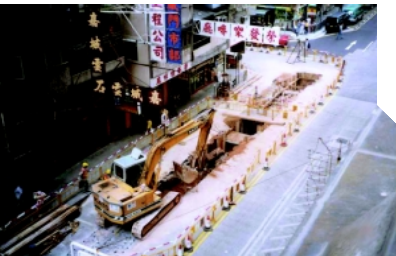
於旺角廣東道與弼街交界興建雨水渠 Construction of stormwater drains at junction of Canton Road and Bute Street, Mong Kok
