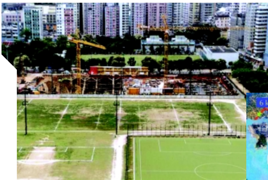
於石硤尾的大坑東遊樂場地下興建蓄洪池 Construction of the underground flood storage tank in progress at Tai Hang Tung Playground, Shek Kip Mei
