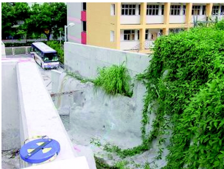
於荃灣麗城花園發業里對上明渠興建防洪牆，以改善該處的排水情況 Flood wall constructed as local drainage improvement works alongside the open channel above Fat Yip Lane, near Belvedere Garden, Tsuen Wan
