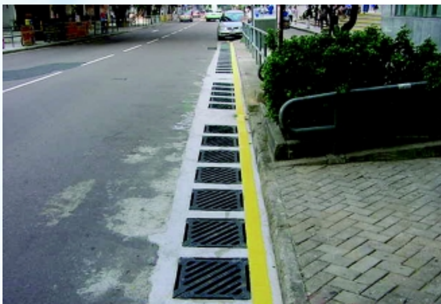
於青山道的截流渠是臨時改善措施的其中部分 Flow interceptor at Castle Peak Road as one of the interim improvement measures
