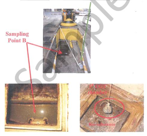
Central Grease Trap B (CGT-B) was located at the entrance of the G/F car park. "Bio-substance" was placed inside the 1<sup>st</sup> chamber of the CGT. Sampling point B was at the outlet of the CGT.
