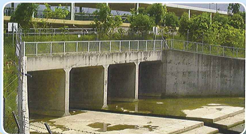
排水道出口 Outlet of a Drainage Culvert
