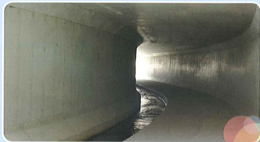
排洪暗渠 Drainage Culvert
