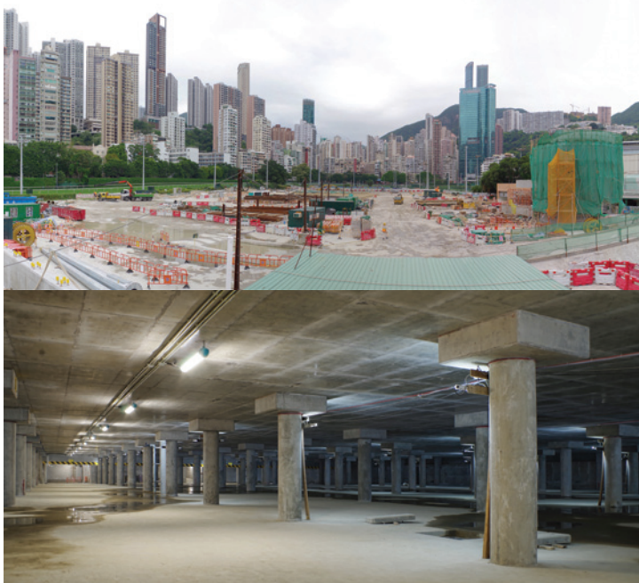
蓄洪池採淺缸設計，只高三米，減少使用水泵抽水機會，節省能源。 A shallow tank of 3-metre high means less water to be pumped out, in order to save power.
