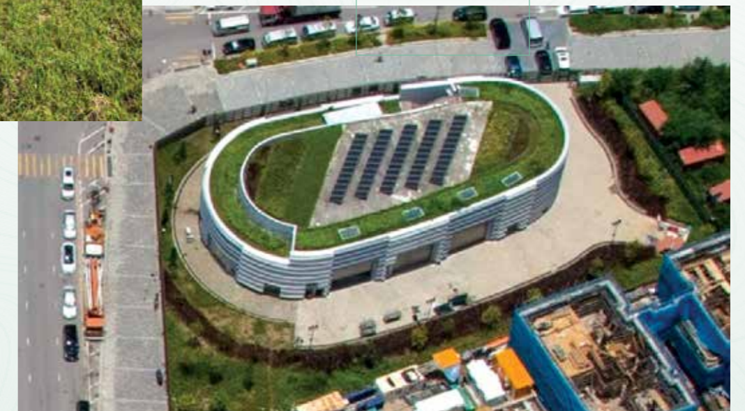
沐泰街污水泵房 Muk Tai Street Sewage Pumping Station
