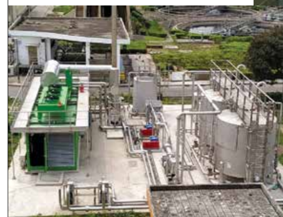
於 2021 年初落成位於大埔污水處理廠的電熱聯供發電系統 Combined heat and power generating system commissioned at Tai Po Sewage Treatment Works in early 2021
