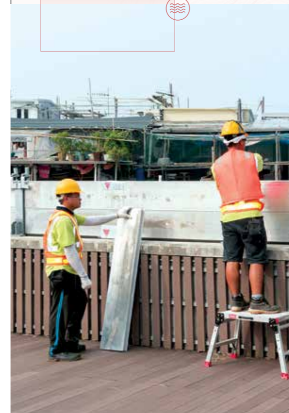
於大澳裝設組合式擋水板 Installing demountable flood barriers in Tai O
