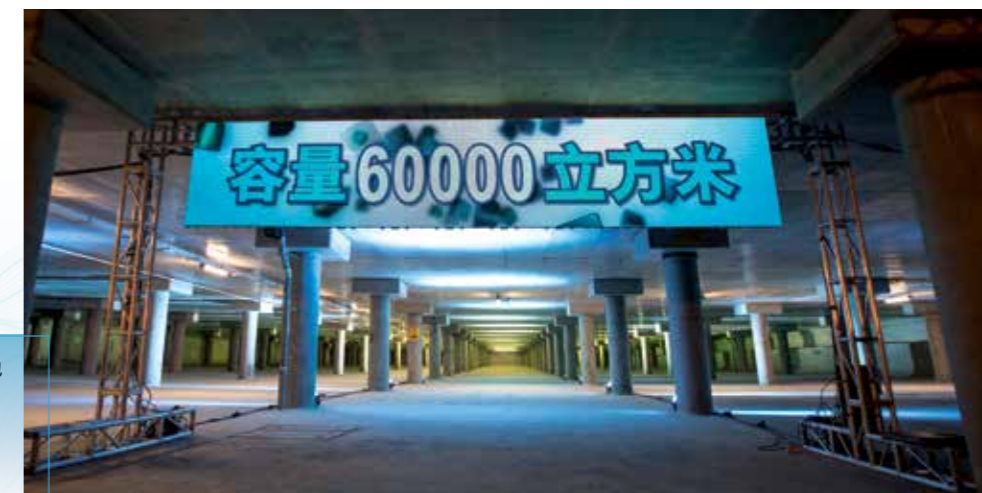
跑馬地地下蓄洪池 Happy Valley Underground Stormwater Storage Tank
