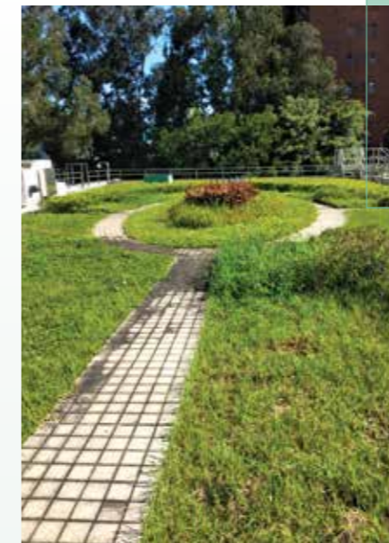
兆康污水泵房 Siu Hong Sewage Pumping Station
