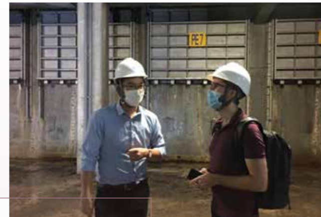
工程師劉耀文先生（左）向記者介紹跑馬地地下蓄洪池 Engineer Mr Alex LAU Yiu-man (left) introduced Happy Valley Underground Stormwater Storage Tank to the reporter
