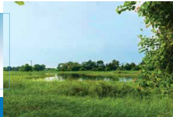
元朗排水繞道人工濕地 Yuen Long Bypass Floodway Engineered Wetland
