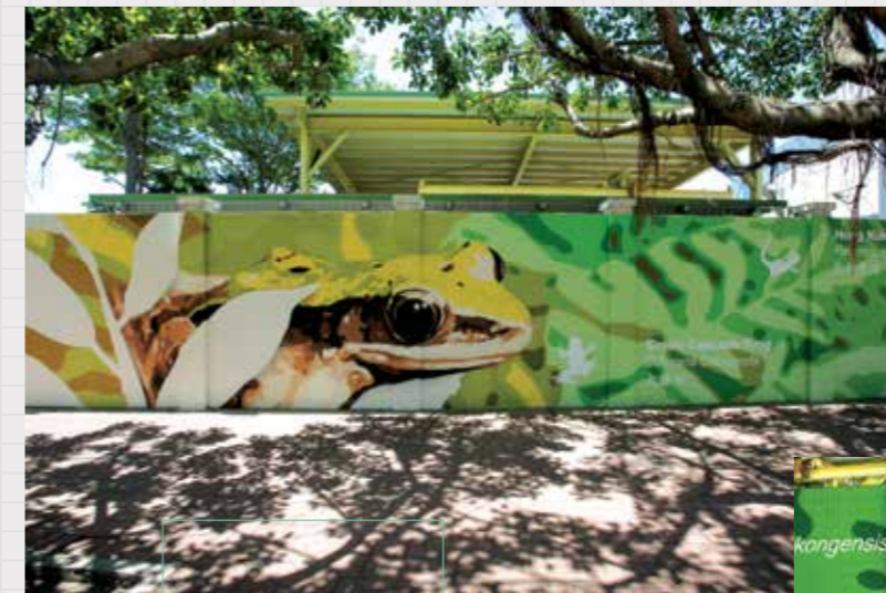
香港機鐵中環污水泵房外牆的藝術作品 Artwork on the walls at Hong Kong Station Central Sewage Pumping Station
