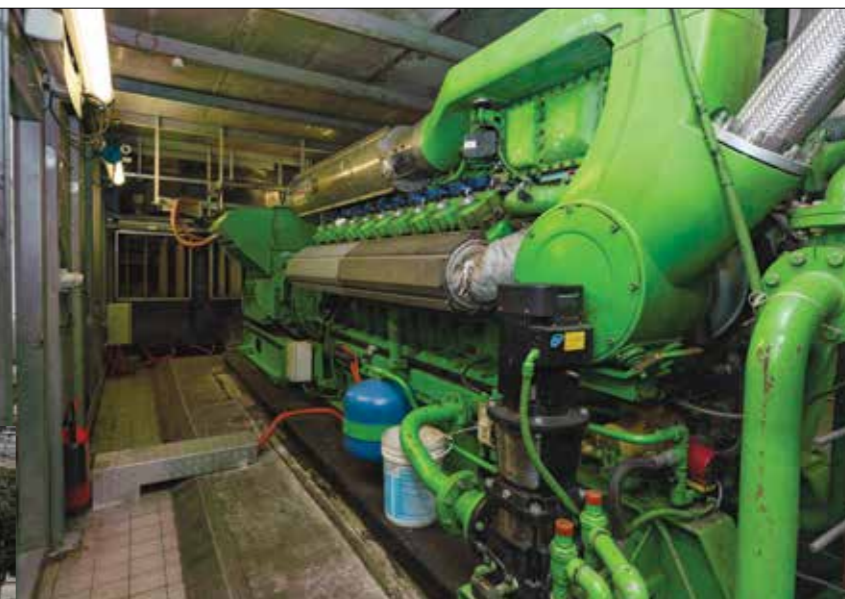
於 2021 年初落成位於大埔污水處理廠的電熱聯供發電系統 Combined heat and power generating system commissioned at Tai Po Sewage Treatment Works in early 2021
