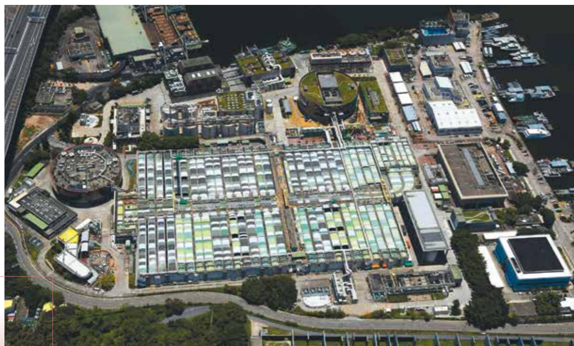
昂船洲污水處理廠 Stonecutters Island Sewage Treatment Works
