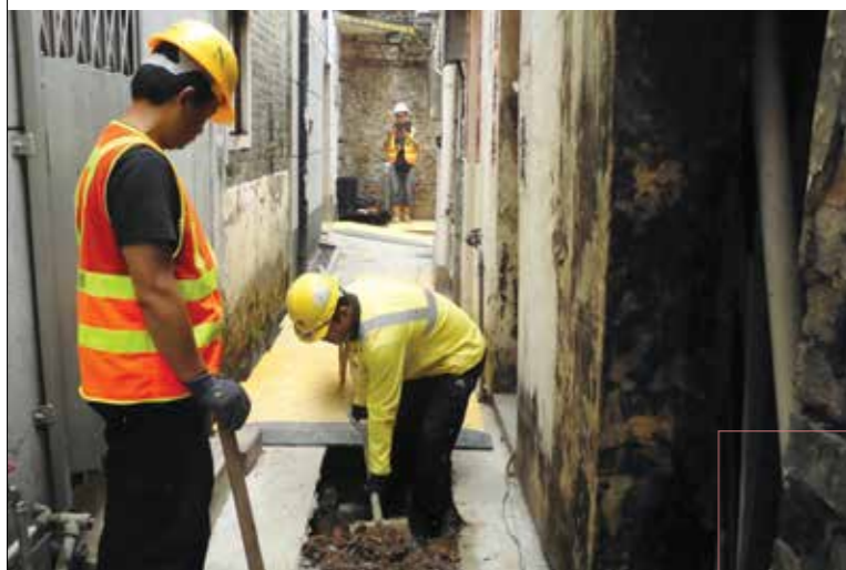
於鄉村敷設污水渠 Sewer laying at a village
