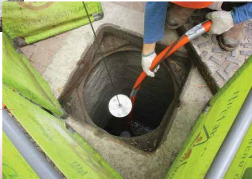
污水沙井修復工程 Sewer manhole rehabilitation works
