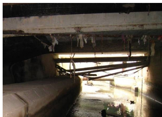
Figure 4 - Existing Utility under Nullah Decking
