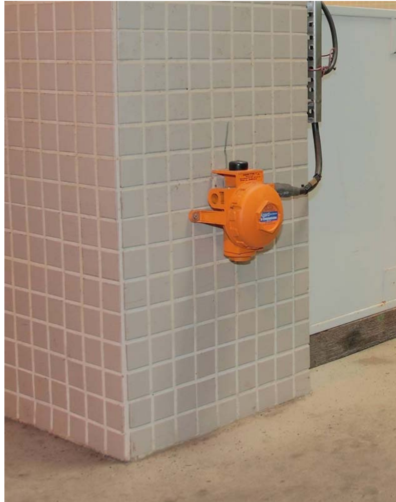
Photo 3: Fixed Type H 2 S Sensor (7 nos.)
