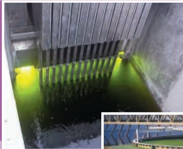
紫外光消毒槽運作中 UV lamps in operation
